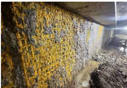
Fig 7: Corrosion Treatment Applied on Exposed Reinforcement
