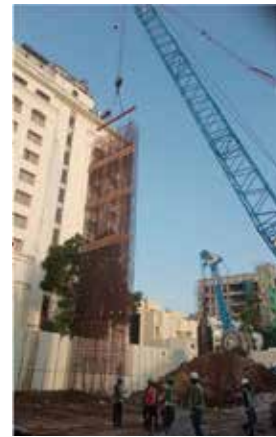
Fig 5: Reinforcement Cage Being Lowered into a D-Wall Panel
