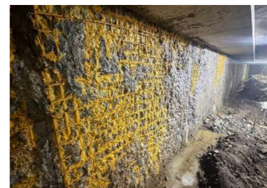
Fig 7: Corrosion Treatment Applied on Exposed Reinforcement
